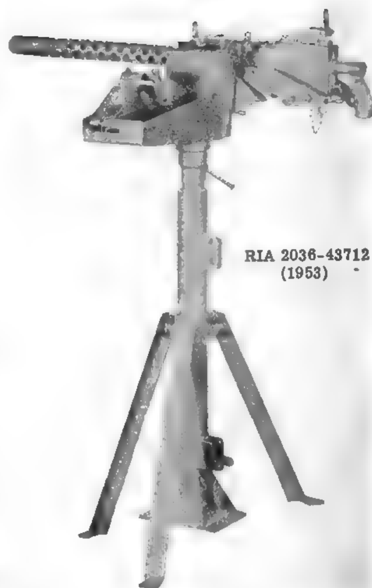
The M31A1 lacked the travel lock that had been furnished with the previous mounts.
